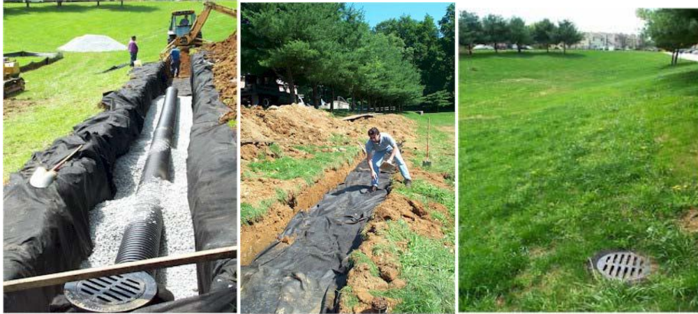
Figure 4: Example of Infiltration Trench Installation
